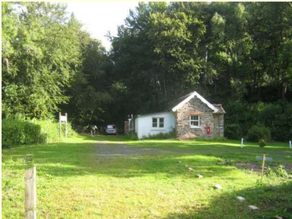
Chelfham Railway Station
